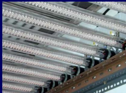
Figure 5. LED arrays mounted inside a CE room
